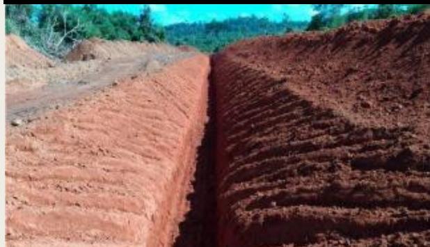
Trenching at the Baldo zone, Cajueiro project
