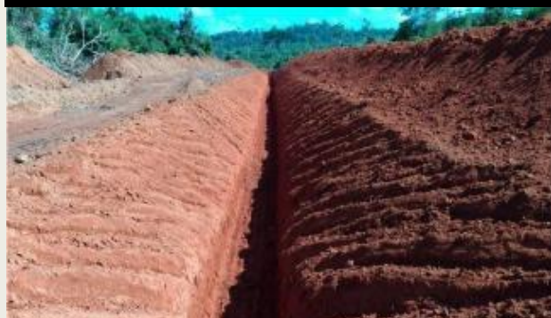
Trenching at the Baldo zone, Cajueiro project
