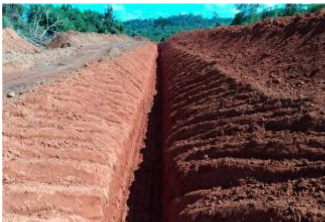
Trenching at the Baldo zone, Cajueiro project
